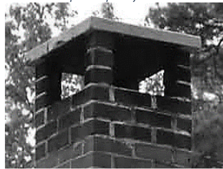
Concrete Cap Chimney Top
