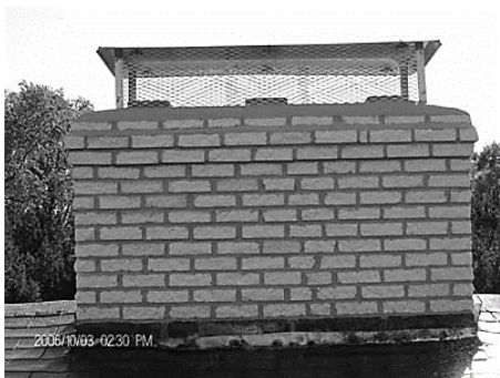
Metal Cap on Clay Liner Chimney Top
